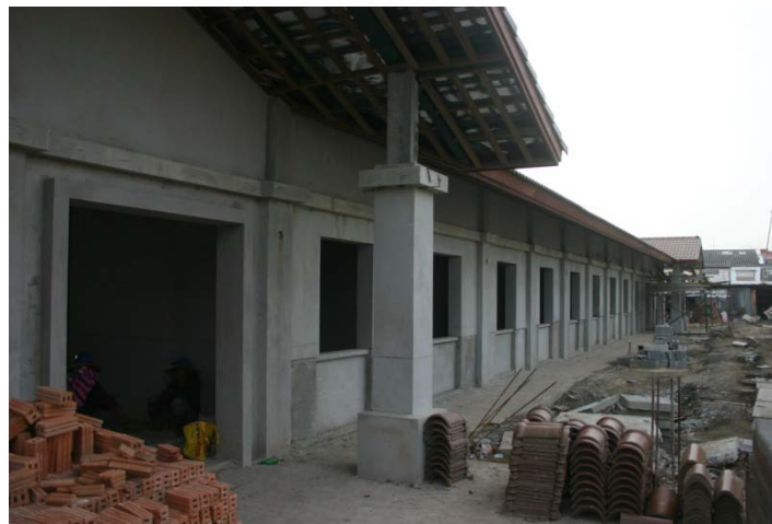
Photo 3 - New building - Classroom Wing
