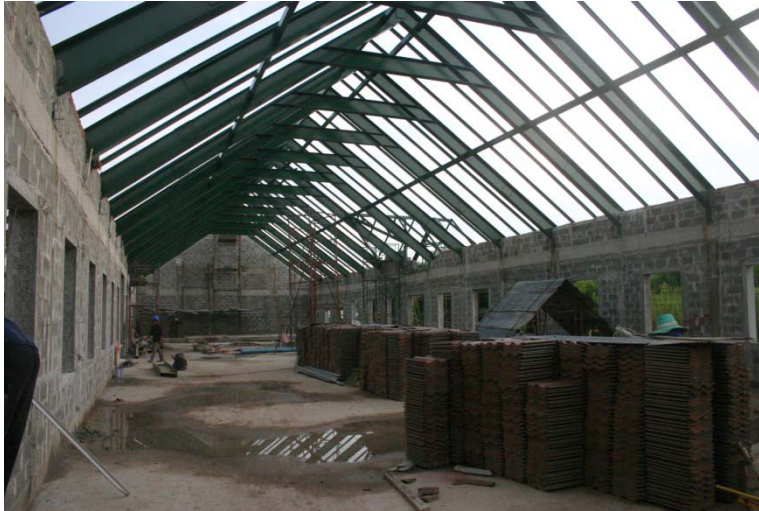
Photo 4 - New building chapel and cultural hall
